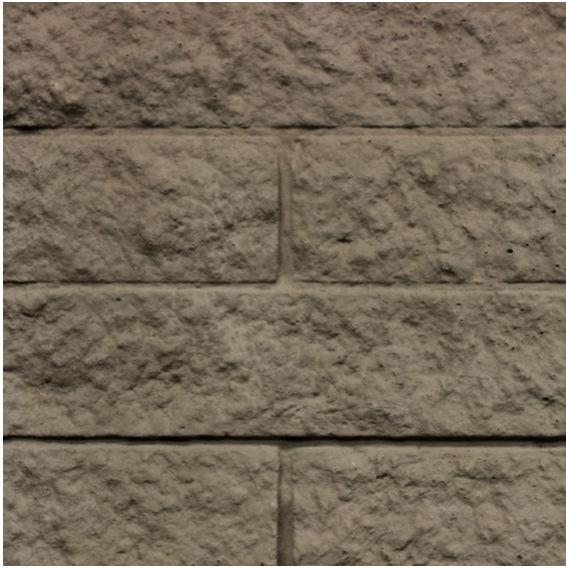
EXTERIOR CLADDING SPLIT FACED CMU: VWP-1B PAINTED 214E PMS 4231C MEDIUM BROWN
