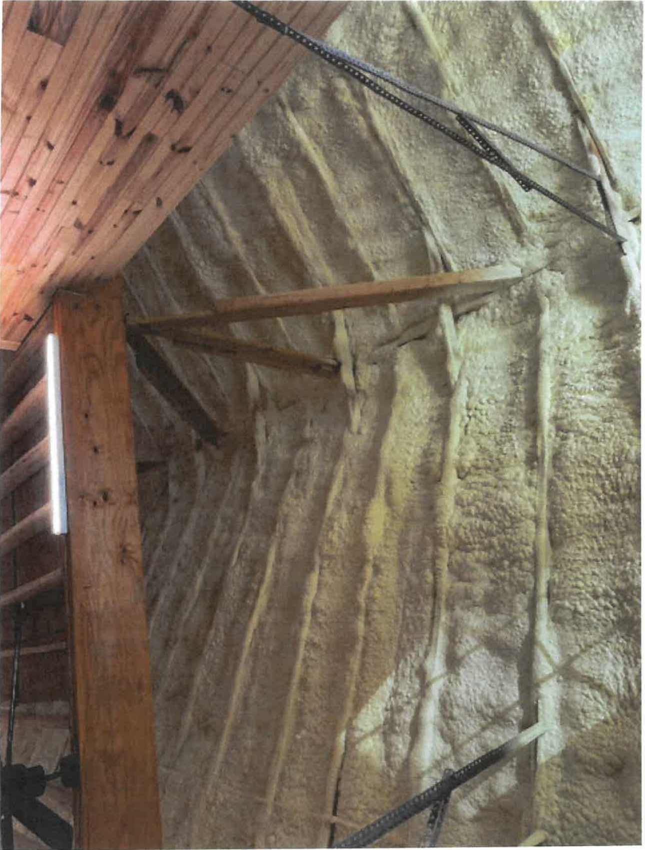
NEW Building 6" spray Foam walls & ceiling
