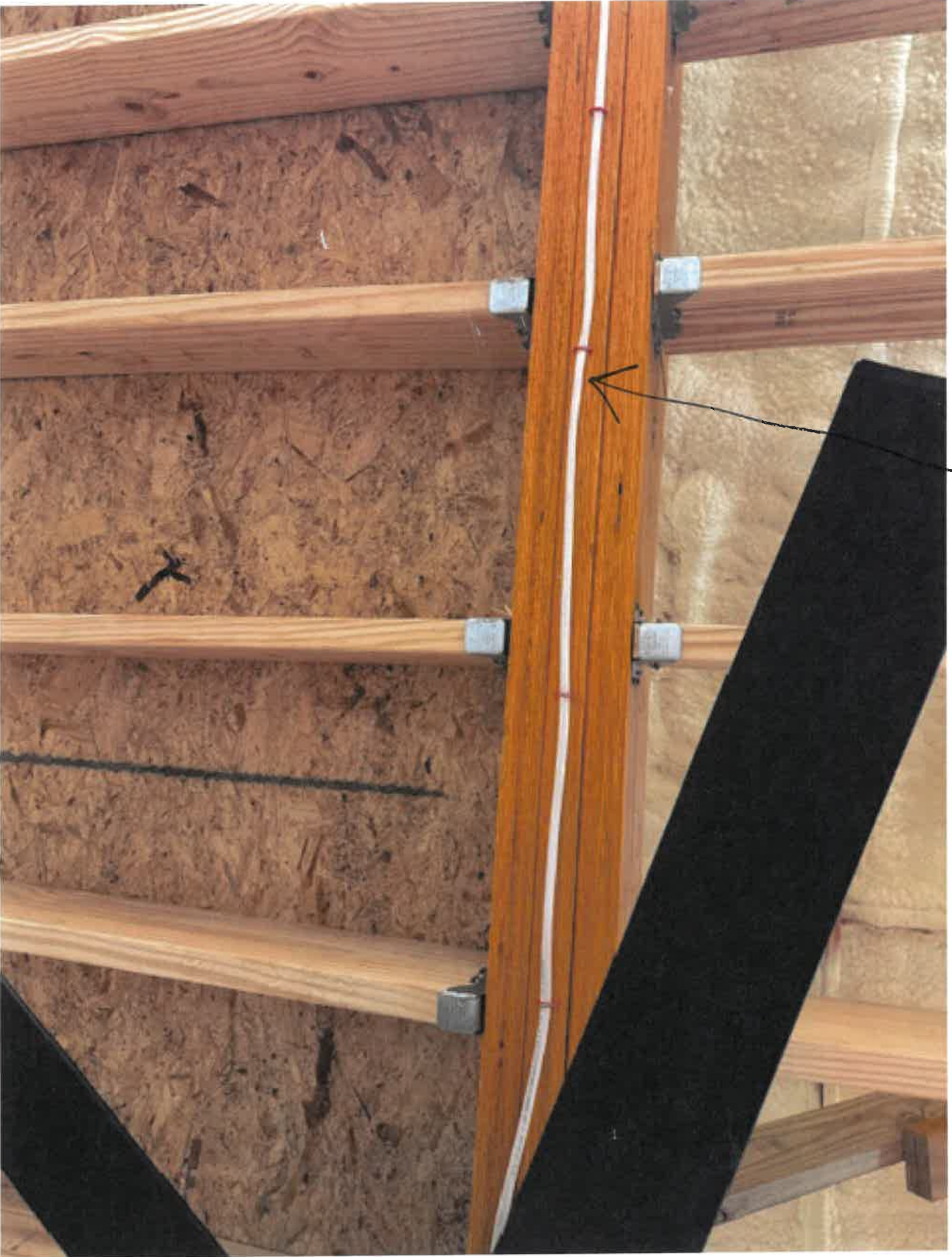
Bottom SHOT OF L.V.L BEAMS
