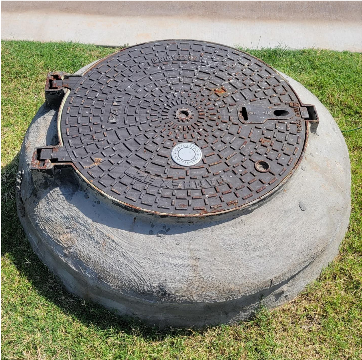
(Image: Manhole at Lucas Retail Addition)
